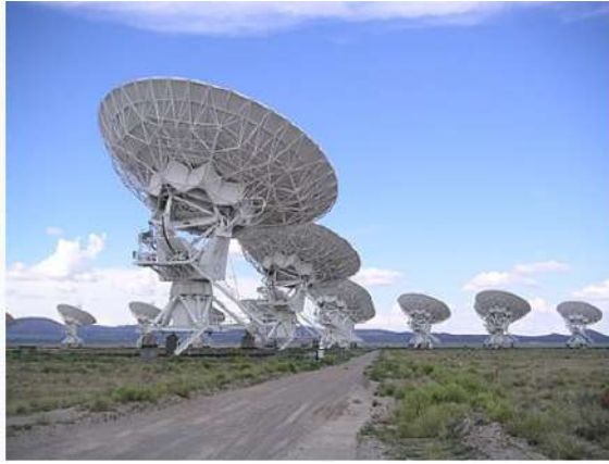
Figure 24.3: Picture of the VLA in New Mexico, USA (Figure by: Wikipedia). The low loss of the circular waveguide gives good SNR according to the fluctuation dissipation theorem [177], which makes the system good for detecting weak radio astronomy signals from outer space.
